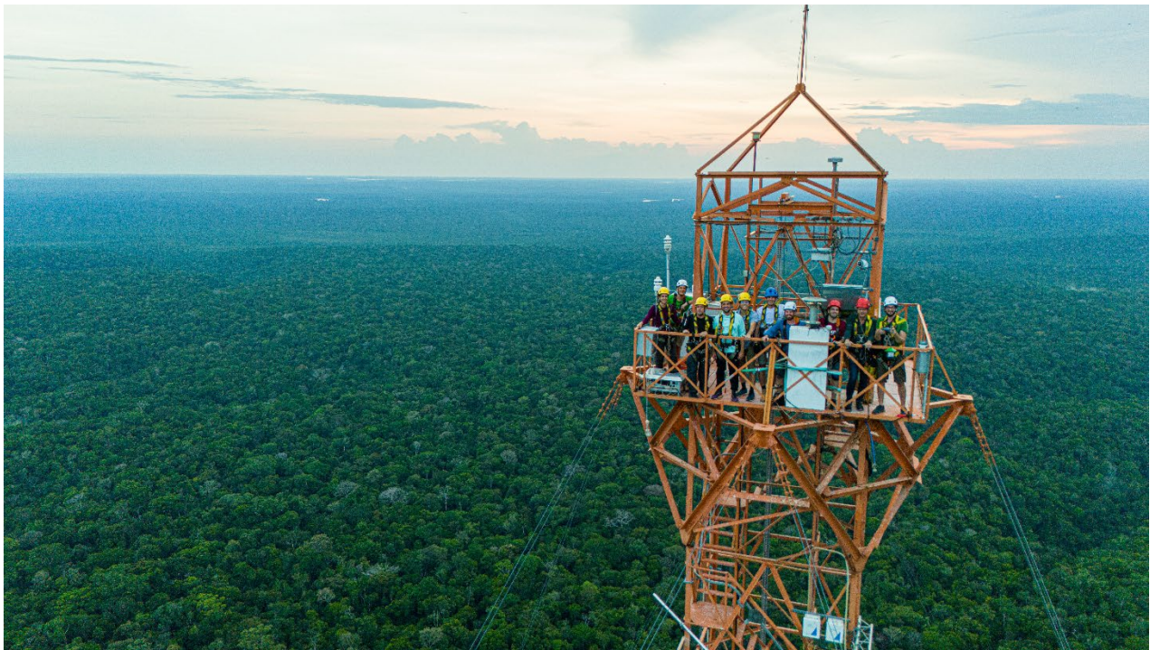
Figure 1. The 325-meter-high tower is the flagship of the Amazon Tall Tower Observatory (ATTO). The tower is equipped with instruments to continuously measure greenhouse gases, reactive gases, aerosols, and energy and water fluxes at various heights.
